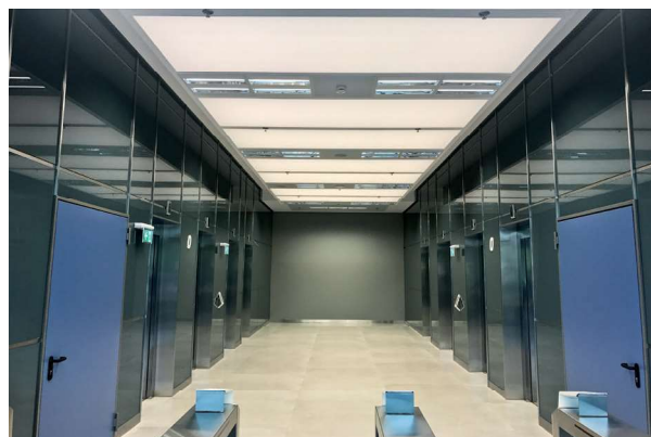
Millenium Center Sofia, Bulgaria – Iluminat interior. Gamele FLAT PANEL, OLOT.
